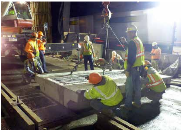
Installation of a WIM site in New York City. Source: NYCDOT.
